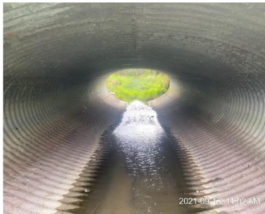
Image 7 – Culvert barrel (looking west)
