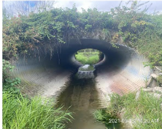
Image 4 – East elevation (looking west)
