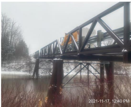
Image 3 - East Elevation (Looking Southwest)
