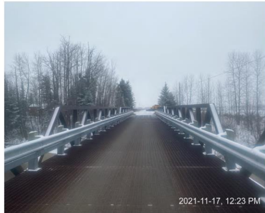
Image 6 - Typical deck grating (looking south)
